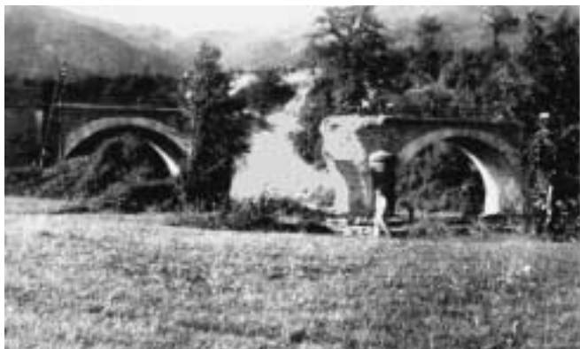
The OSS commandos led by La Gueux destroyed this bridge to delay the movement of Nazi troops in France.
